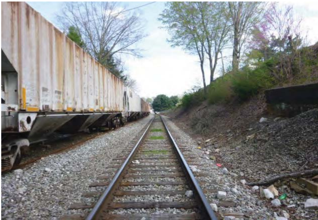
Photo 6: View from Southern Railroad facing east.
