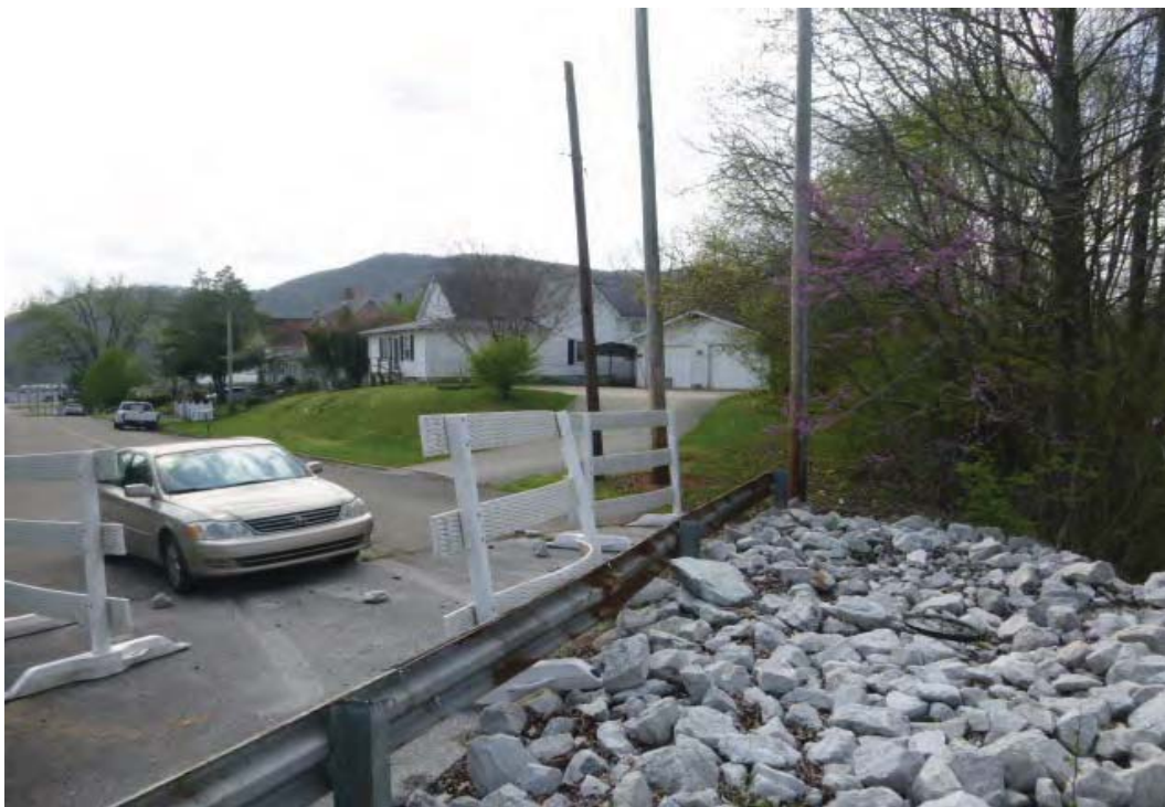
Photo 2. View from south approach facing southwest.
